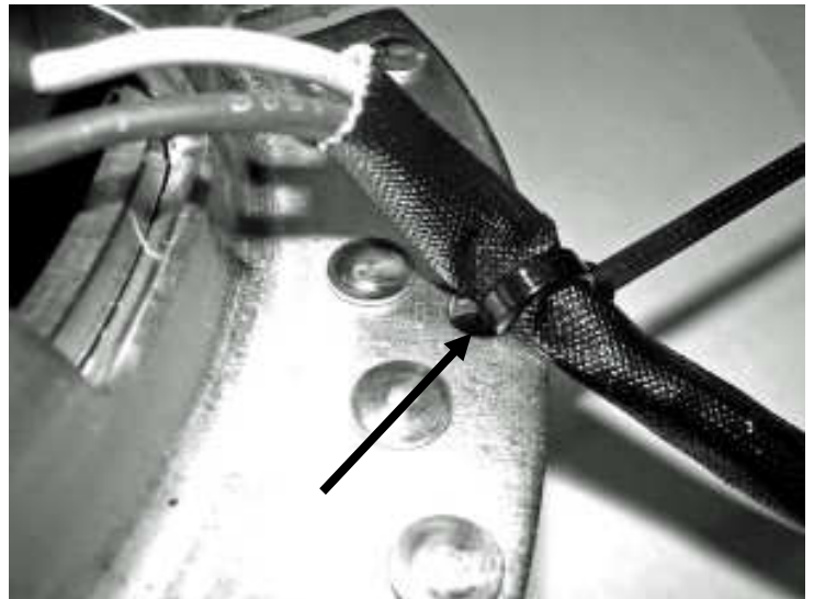
Wire tie prior to installing
